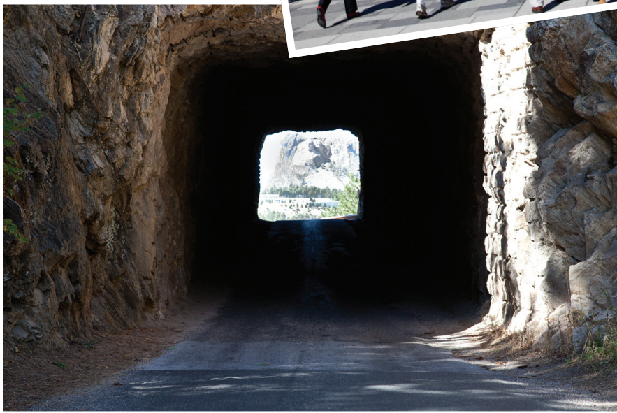
Northbound on US 16 toward Keystone is a scenic road obviously built by the WPA which seems to intentionally traverse the highest points with corkscrew ascents and descents and three of these tunnels, each oriented so as to see the Presidents in the distance.
