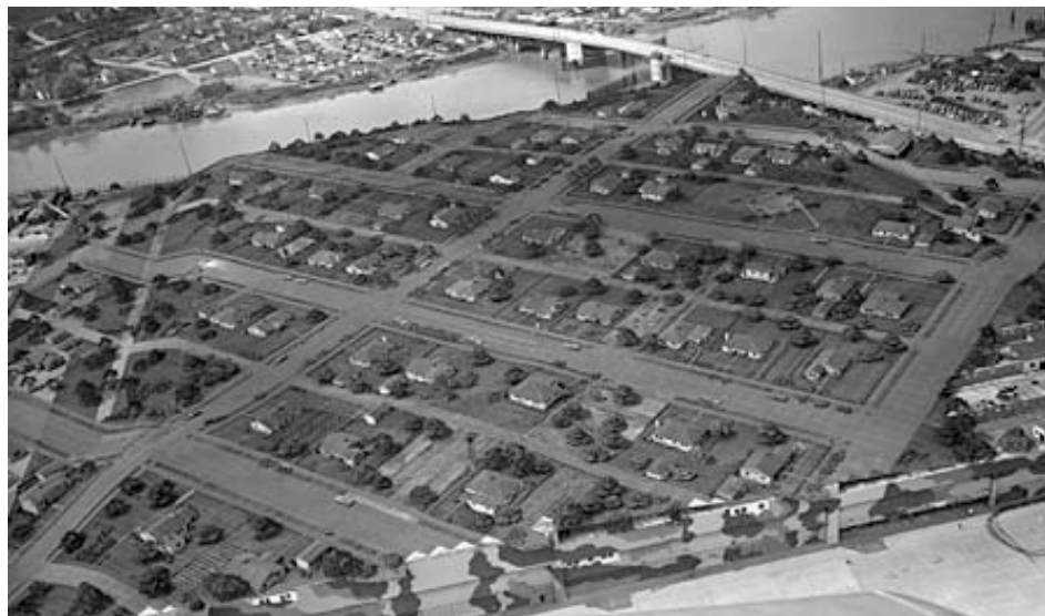
An entire fake town, complete with houses, lawns and trees covered Boeing Aircraft's Plant 2 in Seattle. The design was intended to camouflage the vital defense plant from enemy attack
